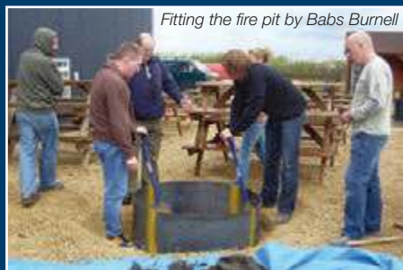
Fitting the fire pit by Babs Burnell
